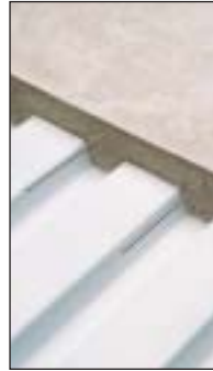
ROOF DECK WITH CONCRETE FLOOR
